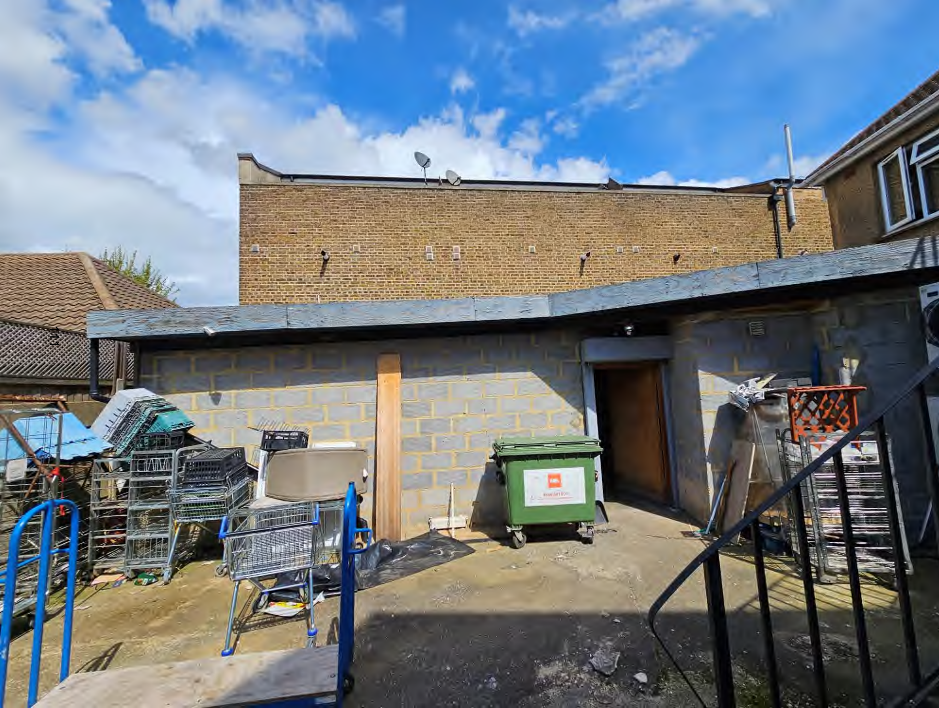
View north to 103 Rochford Road
