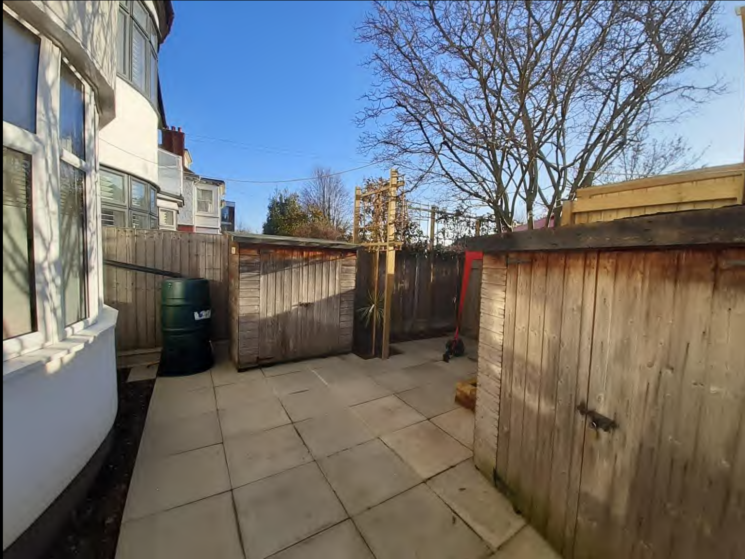
Enclosed area. Sheds are used for storage of prams, maintenance equipment and paraphernalia associated with nursery. Constrc. Manager advised that outbuildings have been on the front part of the site historically.
