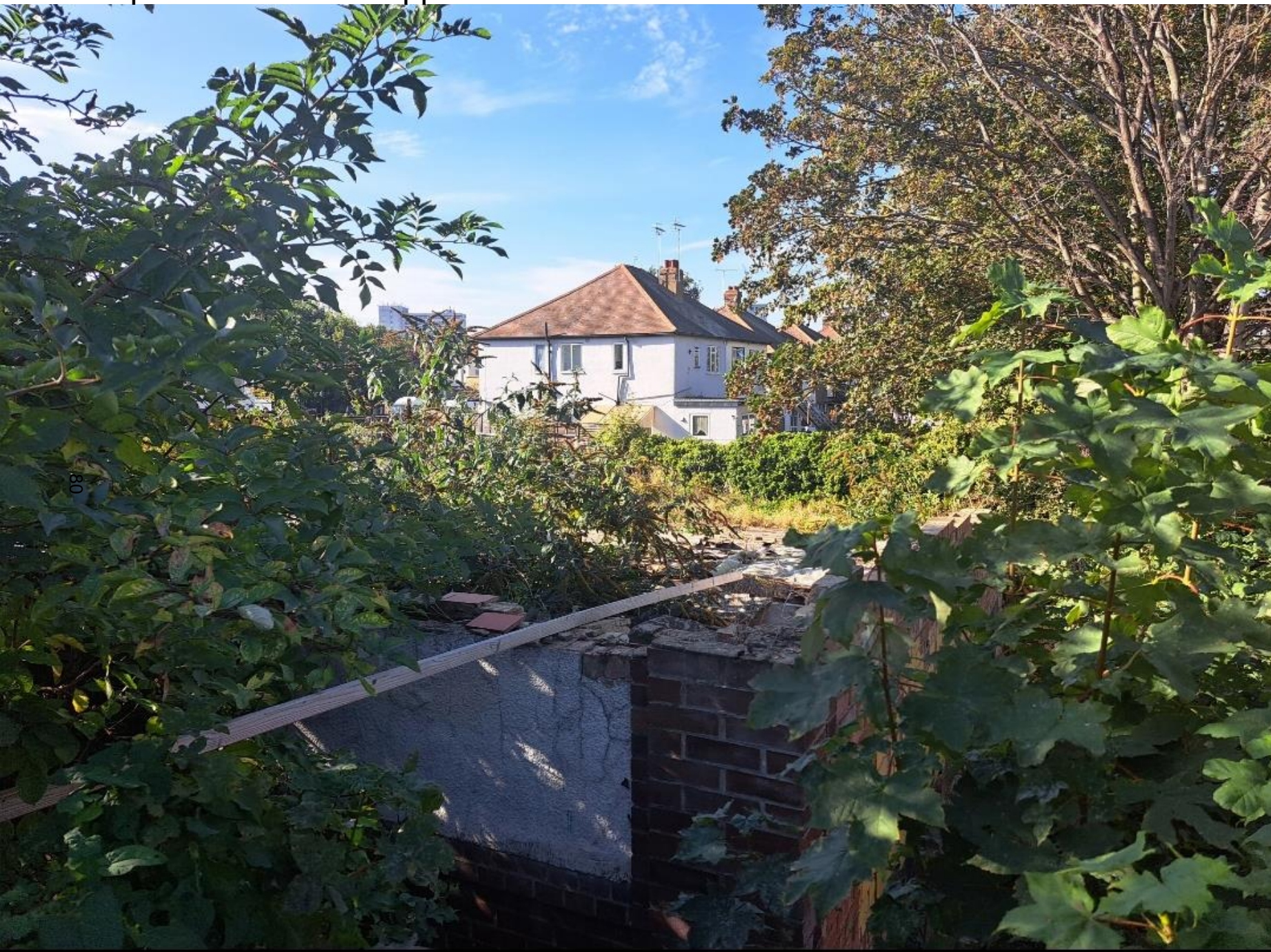
View to poor condition of application site
