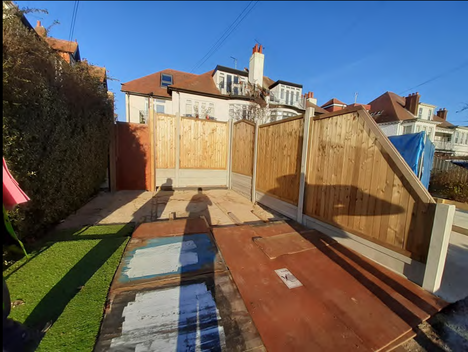
Area to the front of access for the maisonette. Hard standing here is the original surface. Below the fences it is visible by how much the ground was raised.
