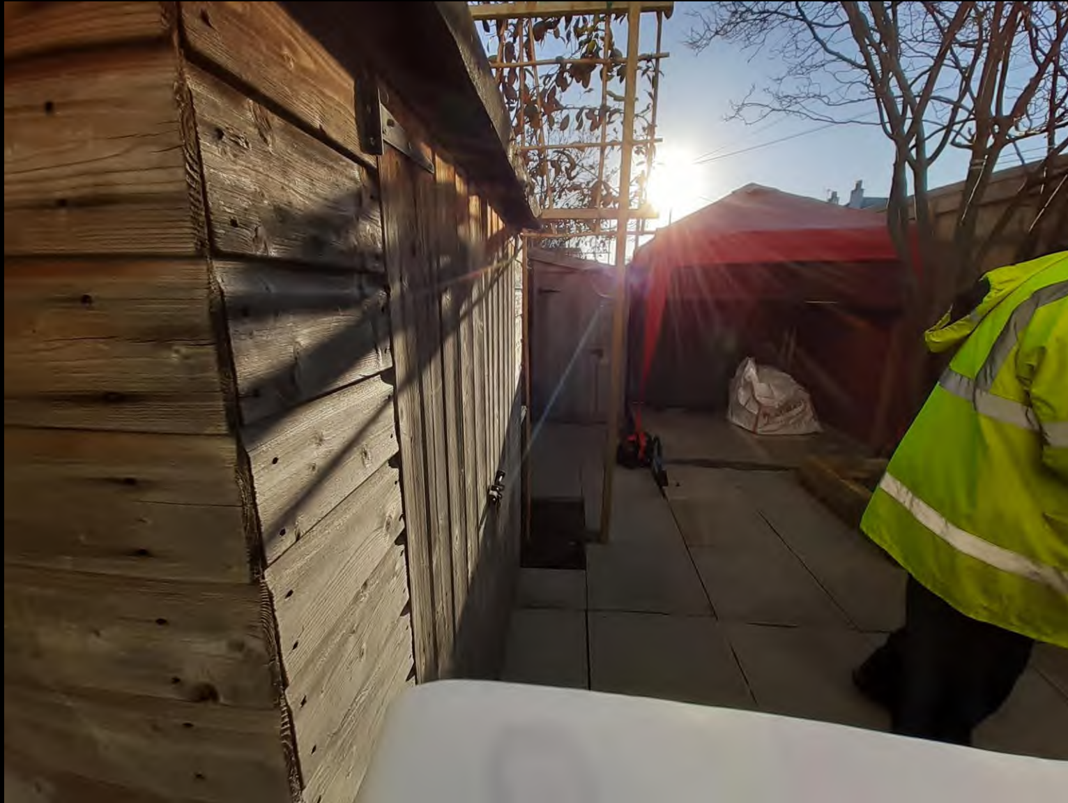
Additional shed and covered area with chattel cover. Used for storage similarly to the other two sheds.
